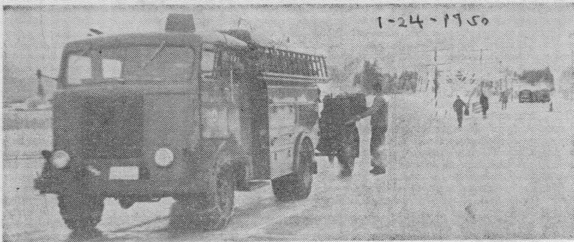
HARD WORK FOR CREWS —January storms with ice and snow have made working conditions in Whatcom county most trying for power and telephone crews. In picture a P. T. & T. truck, with chains on all four wheels, stops to give crewmen a chance to repair ice-covered lines along the Hannegan road.
