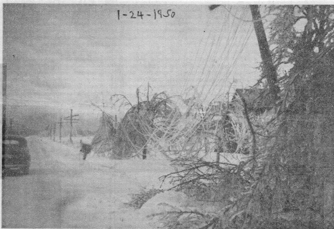
SWINGING LINES —Damage to power and telephone lines in north Whatcom county was heavy last Thursday as the silver thaw struck. Pictured are typical ice conditions on lines along the Everson-Sumas highway, two miles south of Sumas. Note the tree, drooping with ice.
