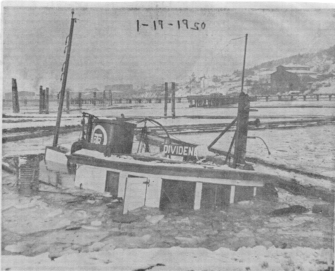
TUG DIVIDEND GOES DOWN —Crunching a hole in its bow when moving ice-jammed logs Wednesday afternoon near the Bellingham Plywood Company, the 65-foot tug Dividend, owned by the Bellingham Tug & Barge Company, sank rapidly. The vessel is pictured down about 100 feet off shore, with no one injured as Skipper John H. Sooter and his three-man crew were taken off by a nearby boat. The Dividend was floated at low tide Wednesday night, pumped out, and taken to drydock Thursday morning at Bellingham Shipyards, Inc. Striking of a submerged object was given as the cause of the accident.—Herald photo.
